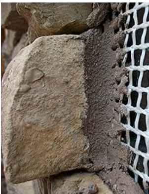
Fig. 1A - Attaching Lath
