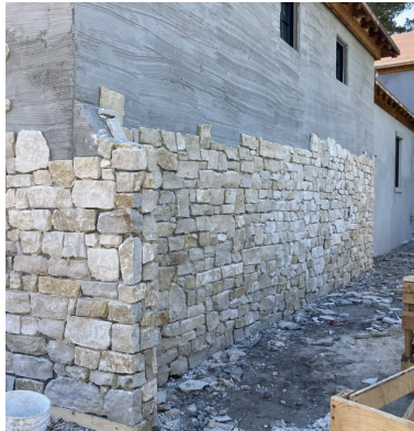
Fig. 1B - Applying scratch coat
